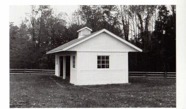
An open air shelter for polo horses turned out to pasture, the loafing shed creates a bold geometry using basic wood elements. The building, measuring  $16 \times 42$  feet, is a straightforward pole structure with wide roof overhangs and a central cupola.
